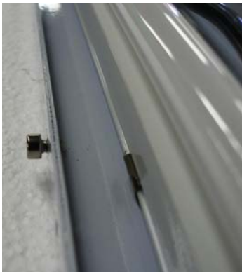
Photo 21: M4 x 6 (Socket) shown with 1/8" (3mm) gap
