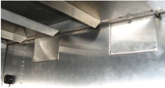
Photo 14: Lamp fixture supports installed
