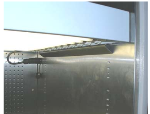
Photo 238: AR canopy seated on top of the support and locked into the center hole.
