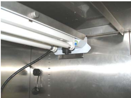
Photo 23: Back Lamp fixture installed (Notice the Thumb screw at the front)
