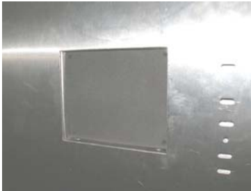
Photo 42: Small insulation installed inside the fan compartment.
