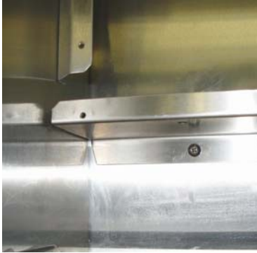
Photo 18: A1000 view after Installing the Back Plenum Bottom Panel
