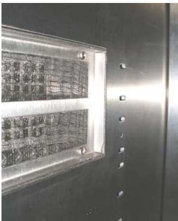
Photo 9: Canopy air inlet filter is showed.
